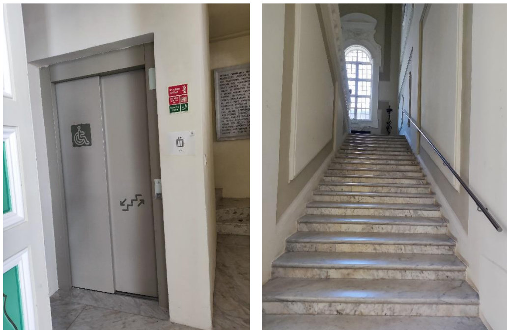
Left: Museum Lift; Right: Museum Stairs with handrail
